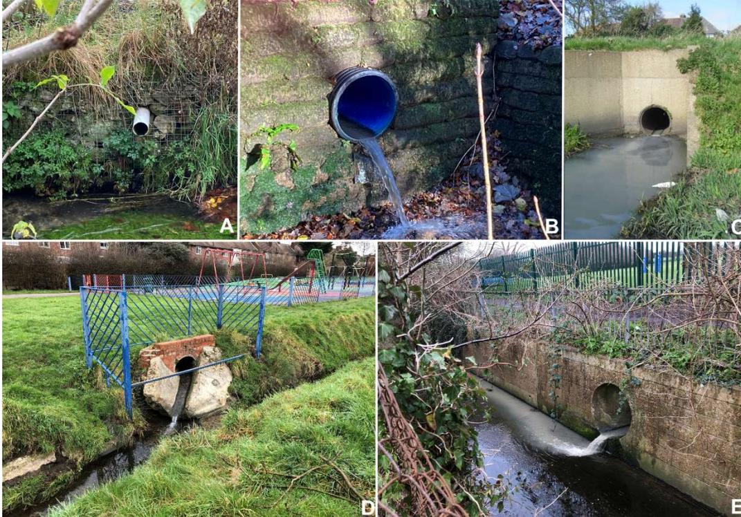
Figure 7. Pipes delivering clear (D), coloured (grey tinge) (B), translucent (C) and opaque (E) water to the river.
