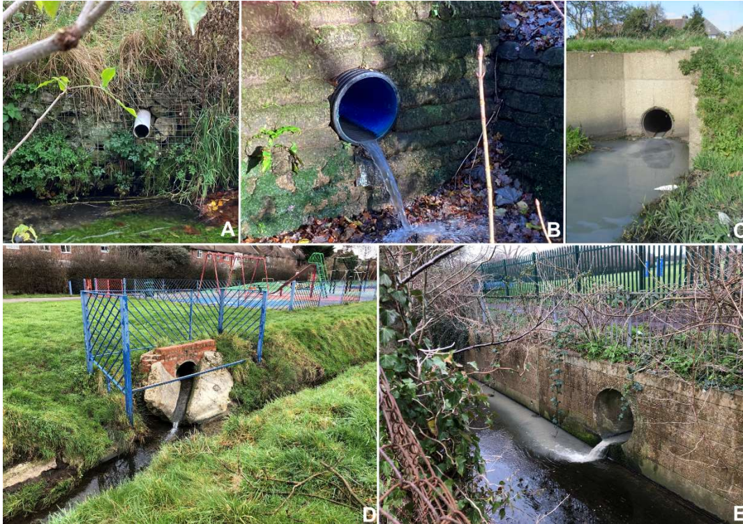
Figure 6. Pipes delivering clear (D), coloured (grey tinge) (B), translucent (C) and opaque (E) water to the river.
