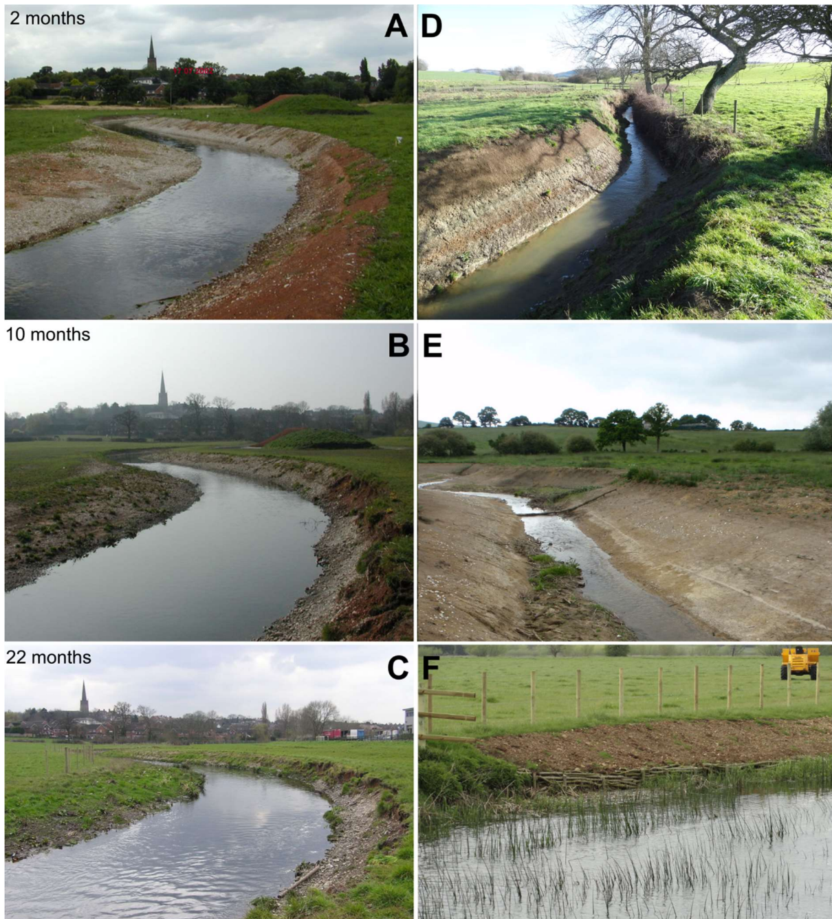
Figure 3: River banks artificially reprofiled (earthworks/dredging). D and E show one or two river banks less than a month after earth works, whereas F shows reprofiling that has just been completed. A, B and C show the same location 2, 10 and 22 months after bank reprofiling has been completed and illustrate that you need to record what you see. Whereas the artificial nature of the exposed banks is clear after 2 months, by 10 months the bare bank on the left still looks artificial but the one on the right is showing the irregular form of a naturally eroding bank, and by 22 months only the bank on the right is bare, it appears to be displaying natural erosion and so should be recorded as natural bank erosion. The photographs were all taken when the river flow was low and so none of the photographs show muddy water in the river next to (i.e. entering the river from) the eroding banks.
